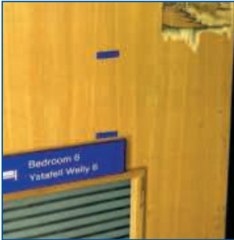
Typical damage caused when a double swing door is forced — Protector in place
